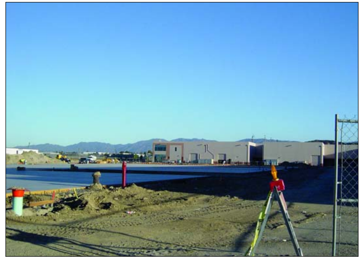
3Pouring the foundation Tilt-up construction begins with the foundation, mid 2005
