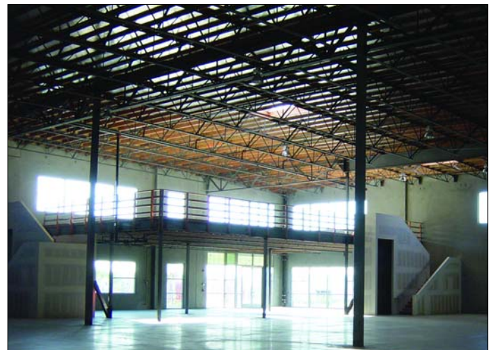
Building "shell" is complete Jan 2006 - outside is done, internal construction begins
